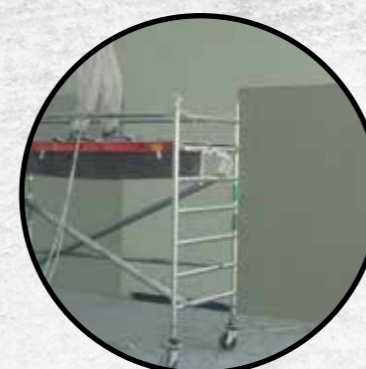
Dry fall NOXYDE® spray turns to powder before hitting the ground
